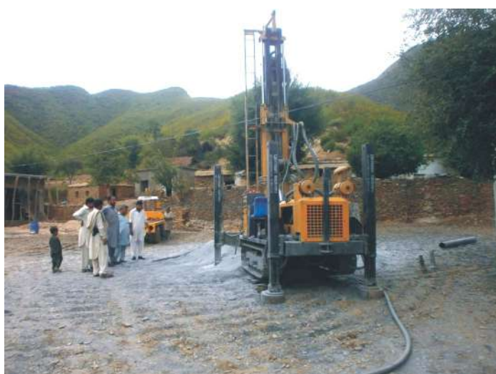
Pic 15: Water Bore Drilling Process in Prrang Dara community
